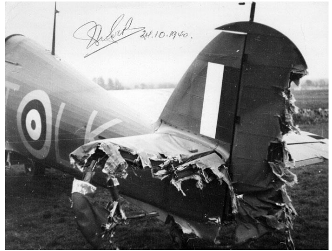
The 87SQN Hurricane that Cock flew on 24 October 1940 showing the badly damaged tailplane after his collision with another aircraft. www.bbm.org.uk
